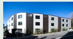
Prime Maison DAIKANYAMA (Meguro-ku, Tokyo) 27 units <Completed in Jan. 2017>
