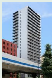
Prime Maison SHIROKANEDAI TOWER (Shinagawa-ku, Tokyo) 220 units <Completed in May 2016>
