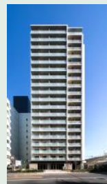
Prime Maison OTSUKA (Toshima-ku, Tokyo) 144 units <Completed in Jan. 2017>
