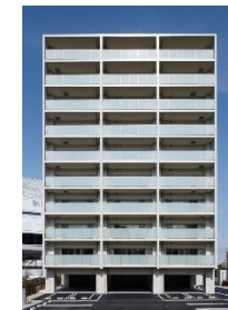
Granmast KAYABA (Nagoya-shi, Aichi) 27 units in total <Completed in Feb. 2012>
