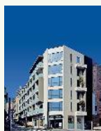
Prime Maison SHINAGAWA (Shinagawa-ku, Tokyo)
