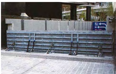
Electrically operated waterproof panel
