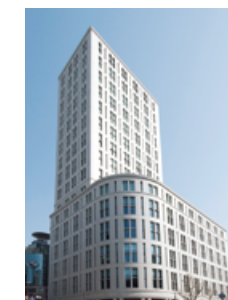
Hommachi Garden City (Office building portion)
